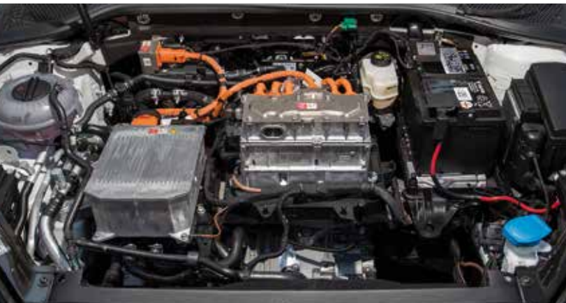
View of the engine bay of the e-Golf
